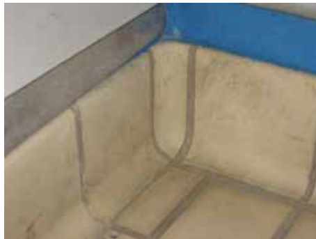
Detail of a hygienic floor with coved corners
